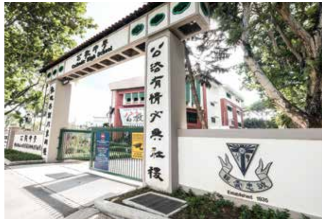
01 CATHOLIC HIGH SCHOOL 9 Bishan Street 22, Singapore 579767
